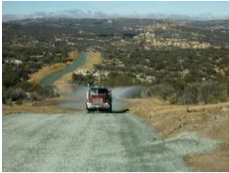
Photo 1: In accordance with MM-BIO-4a and MM-AQ-1, water trucks were diligent in watering down commonly used access roads along the underground alignment.
