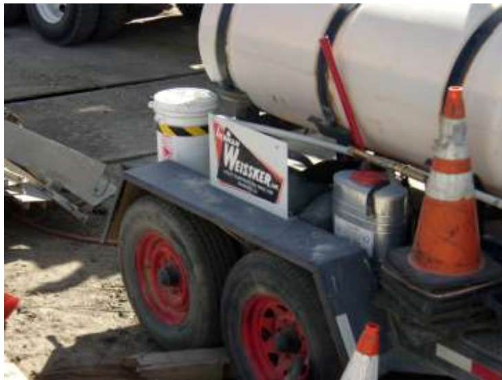
Photo 2: Spill kits were stationed onsite and easily accessible in accordance with MM-HAZ-1a.
